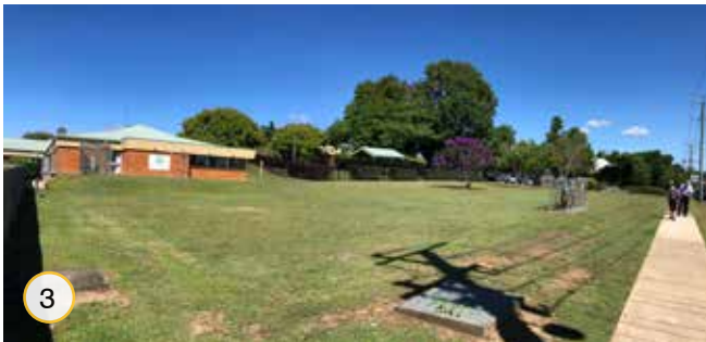
The existing Bundaleer facility on Johnstone Street (Site B) has an extremely deep setback (about 26 metres at this point), set to grass which ties in visually with the school grounds. While the building is set on a slight rise, there is little impact on the streetscape – rather, the combination of setback and single storey height fit well with the neighbourhood.
