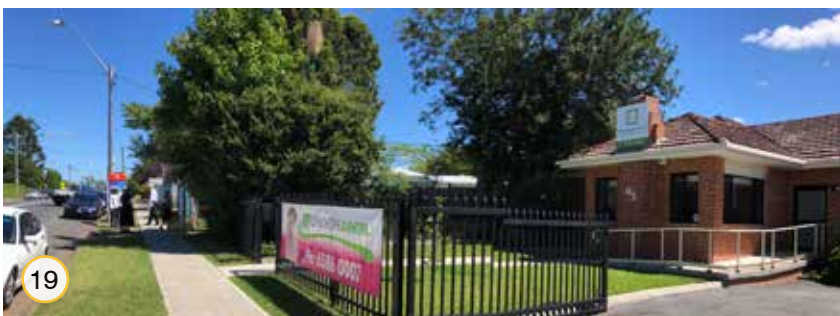
Adjacent to the site, Wauchope Dental is typical of local neighbourhood modifications to make a dwelling house suitable for commercial use: formed driveway, ramp to the entry, signage and formal front fence
