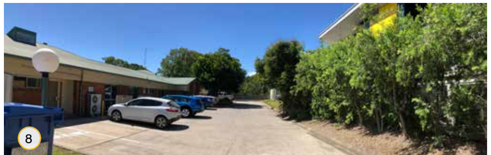
8 A new Hospital palliative care unit is located close to the southern boundary of the Bundaleer site. Both buildings are single storey but the Hospital building has a more dominant presence: it is elevated, has higher ceiling heights and high level windows. Patient rooms face north but there are minimal privacy issues due to the back of house / service character of Bundaleer in this location, and screen planting (in a landscape strip on the Bundaleer side)
