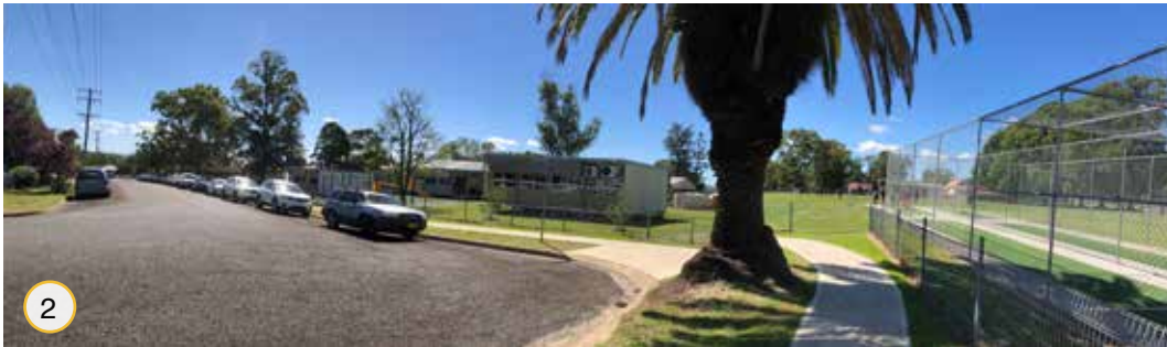
The corner of Johnstone and Mackay Streets, looking north past Wauchope Public School's collection of low-scale prefab classrooms, and east across the school and church grounds within the block. The canary palm, and cricket nets to the right are on axis with the view south down Mackay Street towards part of the existing Bundaleer building.
