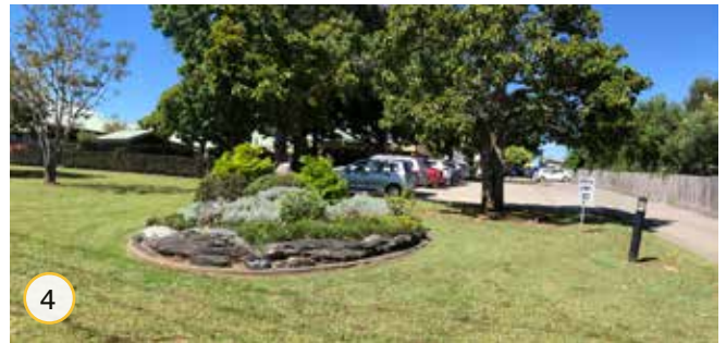
The existing Bundaleer building steps back even further on the western part of its site and almost 'disappears' behind the trees and landscape treatment.
